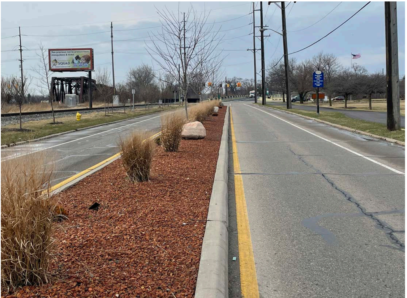
Figure 16: North Dixie Highway median improvement between Noble Avenue and Elm Avenue (Quinn Evans)
